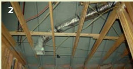
Don't strangle your ducts. Supporting ducts as shown in photo 1 results in a significant loss of air flow. Photo 2 shows a correct installation.
