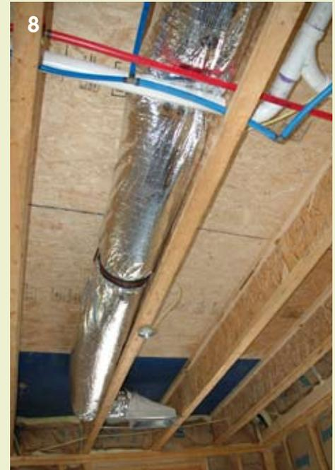
mechanicals. Last, be sure to test for duct leaks. Measuring leakage with a duct blaster is the only sure way to evaluate system leakage.
